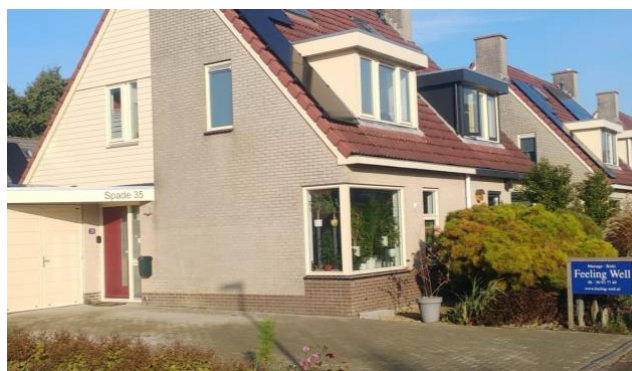
Feeling Well te Wieringerwerf
